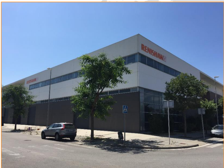
Renishaw Ibérica, S.A.U – new facility in Gavà, near Barcelona
